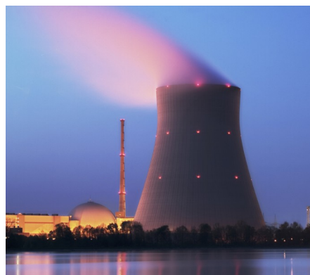
Nuclear power plant
